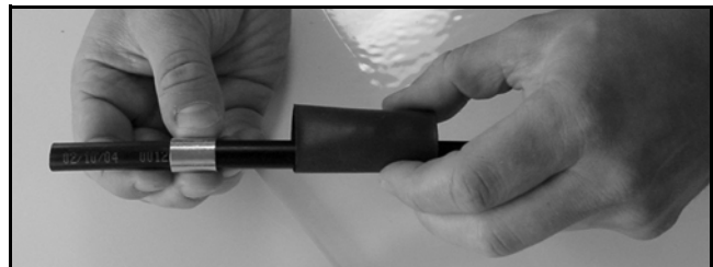
Figure 91: Placing the Heat Shrink Sleeve and Ferrule
