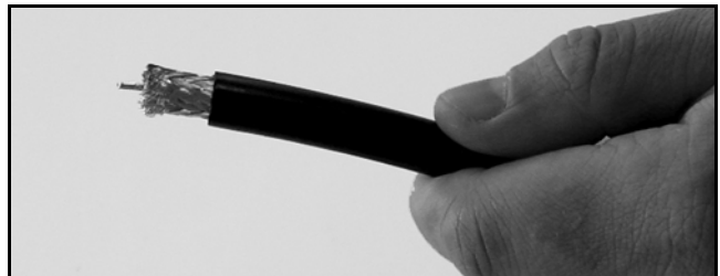
Figure 83: Cable Stripped, Exposing Dielectric
