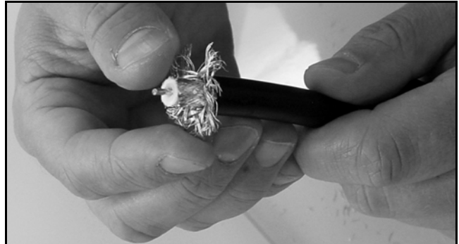
Figure 107: Flaring the Braid
